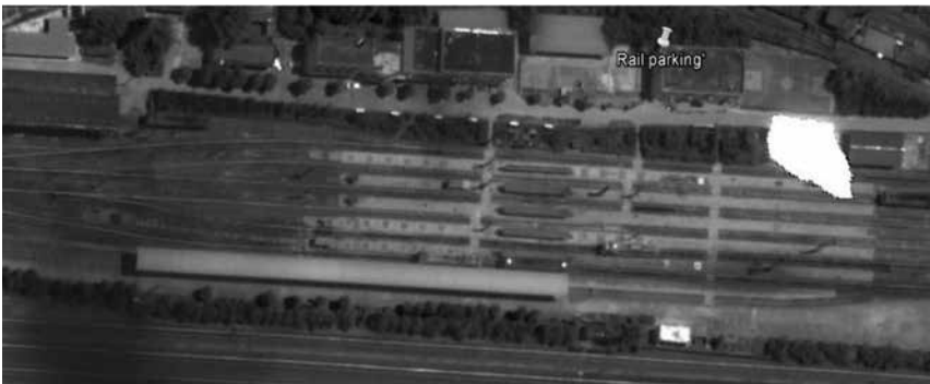
Fig 5: Rail Parking/ Maintenance Garage, Xinyang
