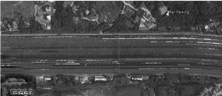
Fig 4: Rail Parking/ Maintenance Garage, Xinyang
