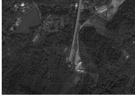
Fig 3: Mountain Tunnel South of Xinyang
